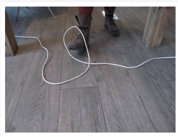
Unsafe: loose extension cords
