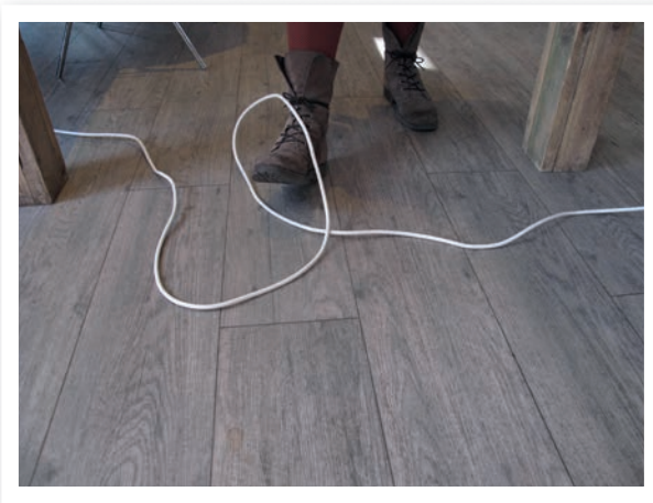
Unsafe: loose extension cords
